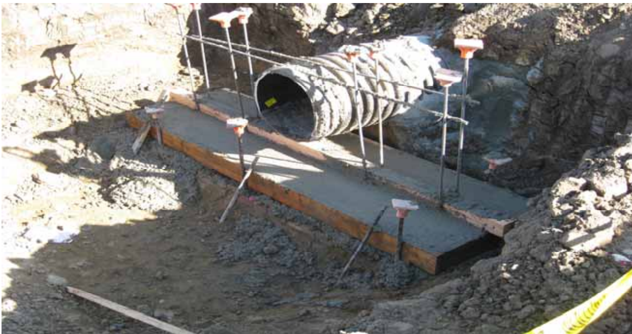
Headwall on Stage 1 Drainage
