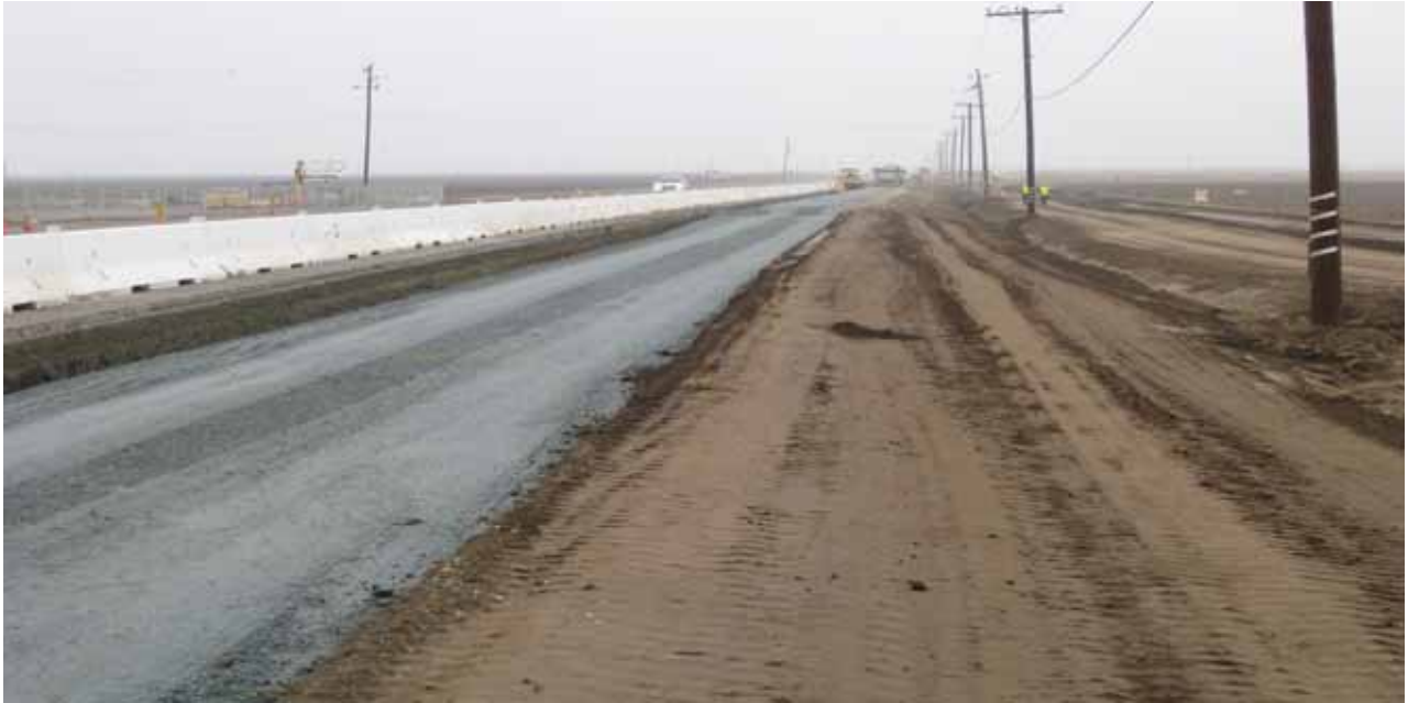
Embankment and Shoulder Widening on Stage 2
