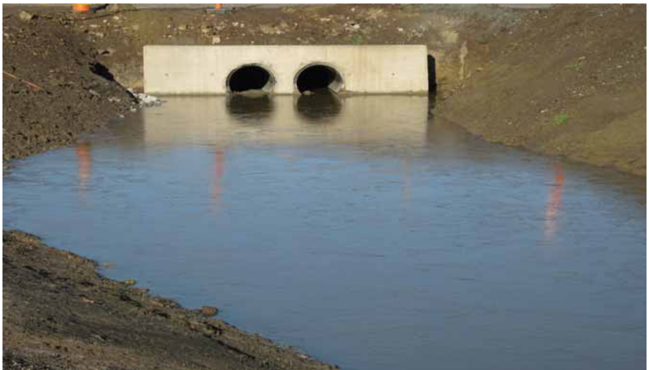
Drainage System at Shore Rd with new Headwal
