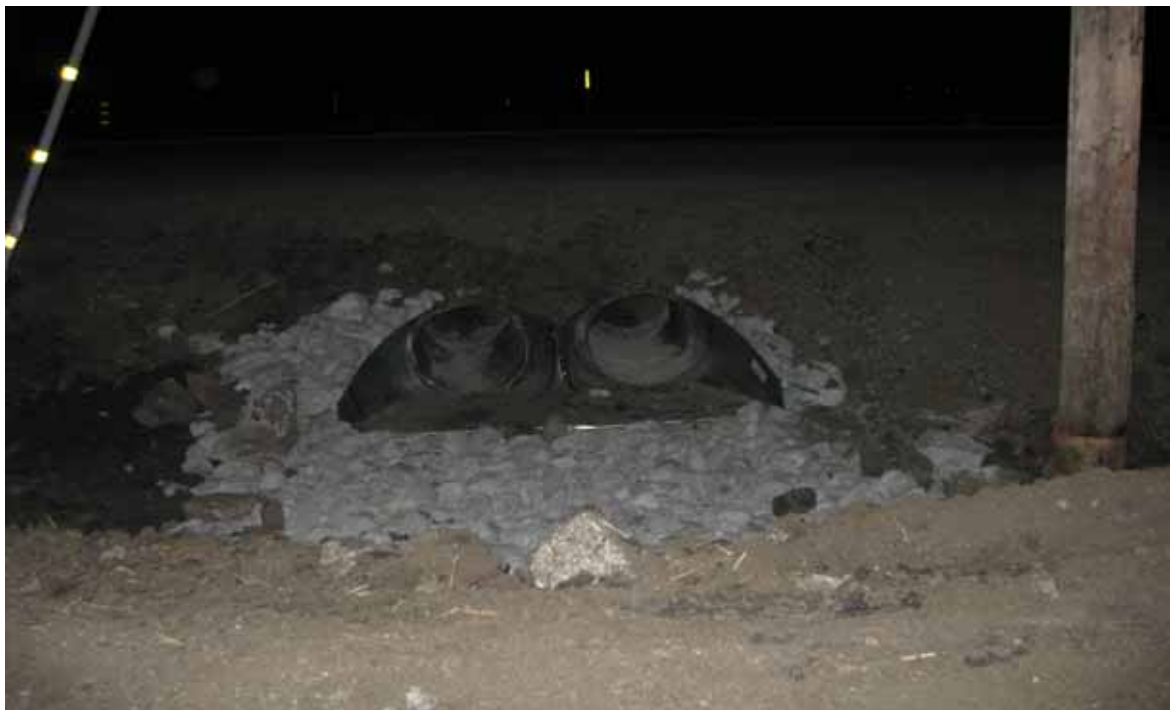
Flared End and RSP drainage Rock on Stage 1
